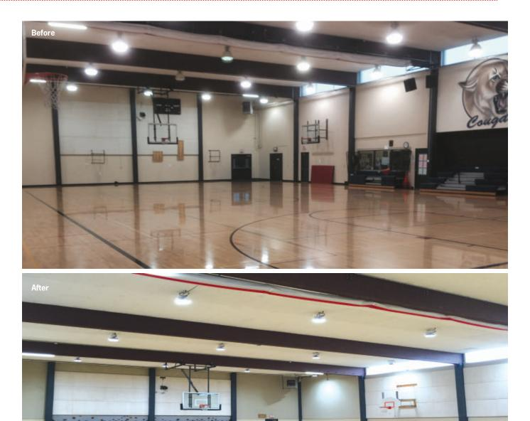
The school's gymnasium went from dingy to bright with the installation of MaxLite's 150W LED round pendant high-bays, which feature narrow beam distribution and deliver more than 16,000 lumens while consuming 60% less energy than the previous metal halides.
