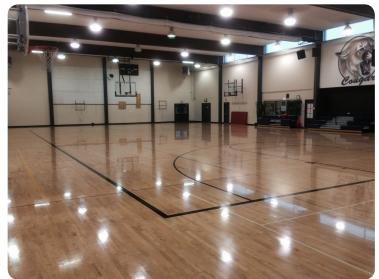
Before: Metal halide fixtures produced glare and required time to warm up.
