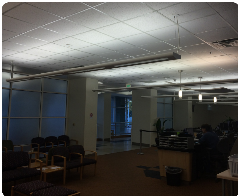
Before: The reception area was unevenly lit by suspension-mounted linear fixtures.
