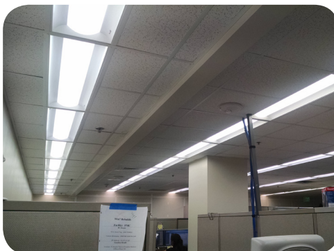
Before: The reception area was unevenly lit by suspension-mounted linear fixtures.
