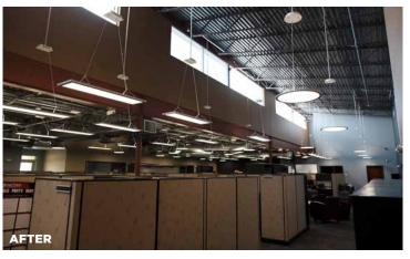
In the open office bullpen, employees complained of low light levels and shadows produced by the existing two-lamp indirect/direct fluorescent pendants. By applying a combination of MaxLite LED Indirect/Direct 1'x4' pendants and 2'x4' round pendants, Red Mountain was able to reduce the fixture count (from 73 to 64) and increase lumens to bring much-needed functional light to work areas. The slim form factors of the pendants also contributed to a more open and airy space.
