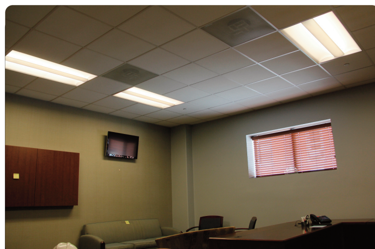
Pictured is Warren Geller's former office with basket-type fluorescent troffers
