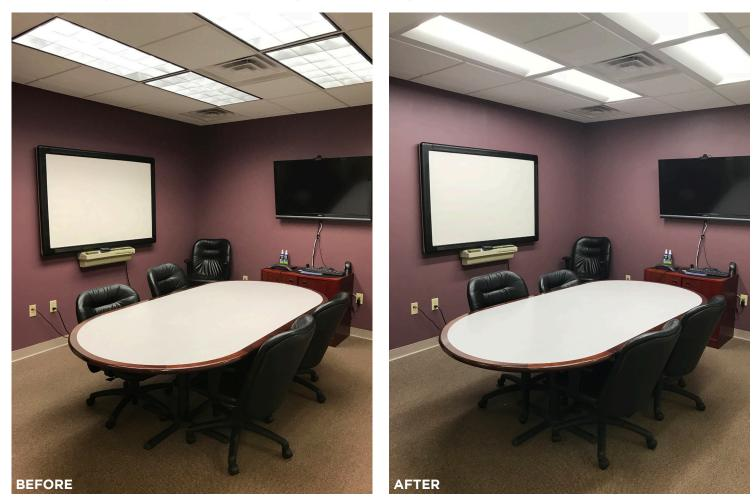
Total wattage for the existing building lighting was approximately 22,496 watts, with calculated usage of 4,351 kWh per month. After the LED retrofit, building lighting is approximately 6,669 watts, with calculated usage of 1,467 kWh/month. By switching to LED, the InSite Group will save 34,608 kWh and \$4,436 in energy and maintenance costs annually.
