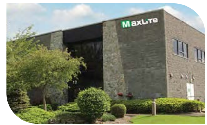
(HQ) West Caldwell, NJ
