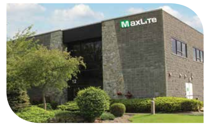
(HQ) West Caldwell, NJ
