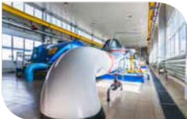
WASTE WATER TREATMENT
