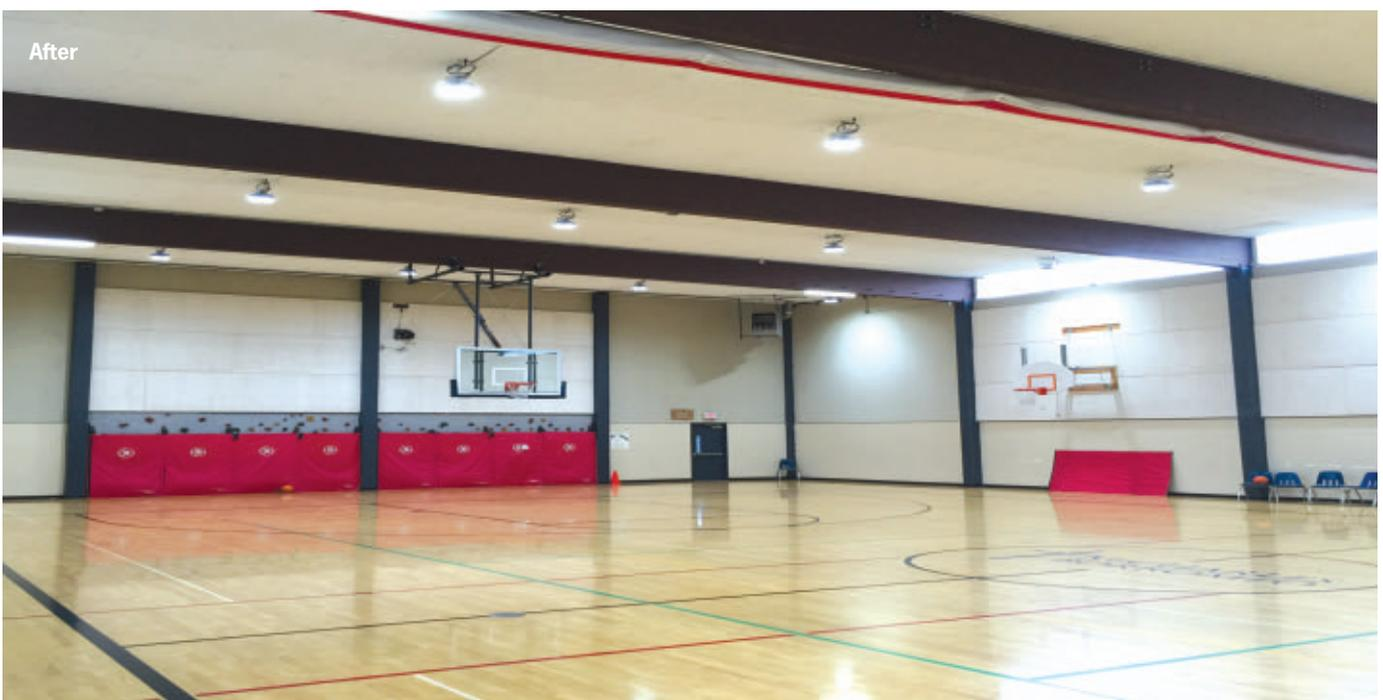
The school's gymnasium went from dingy to bright with the installation of MaxLite's 150W LED round pendant high-bays, which feature narrow beam distribution and deliver more than 16,000 lumens while consuming 60% less energy than the previous metal halides.
